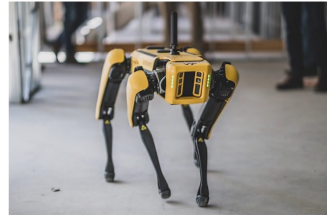
Boston Dynamics robot dog used to inspect construction work at Virginia Tech
